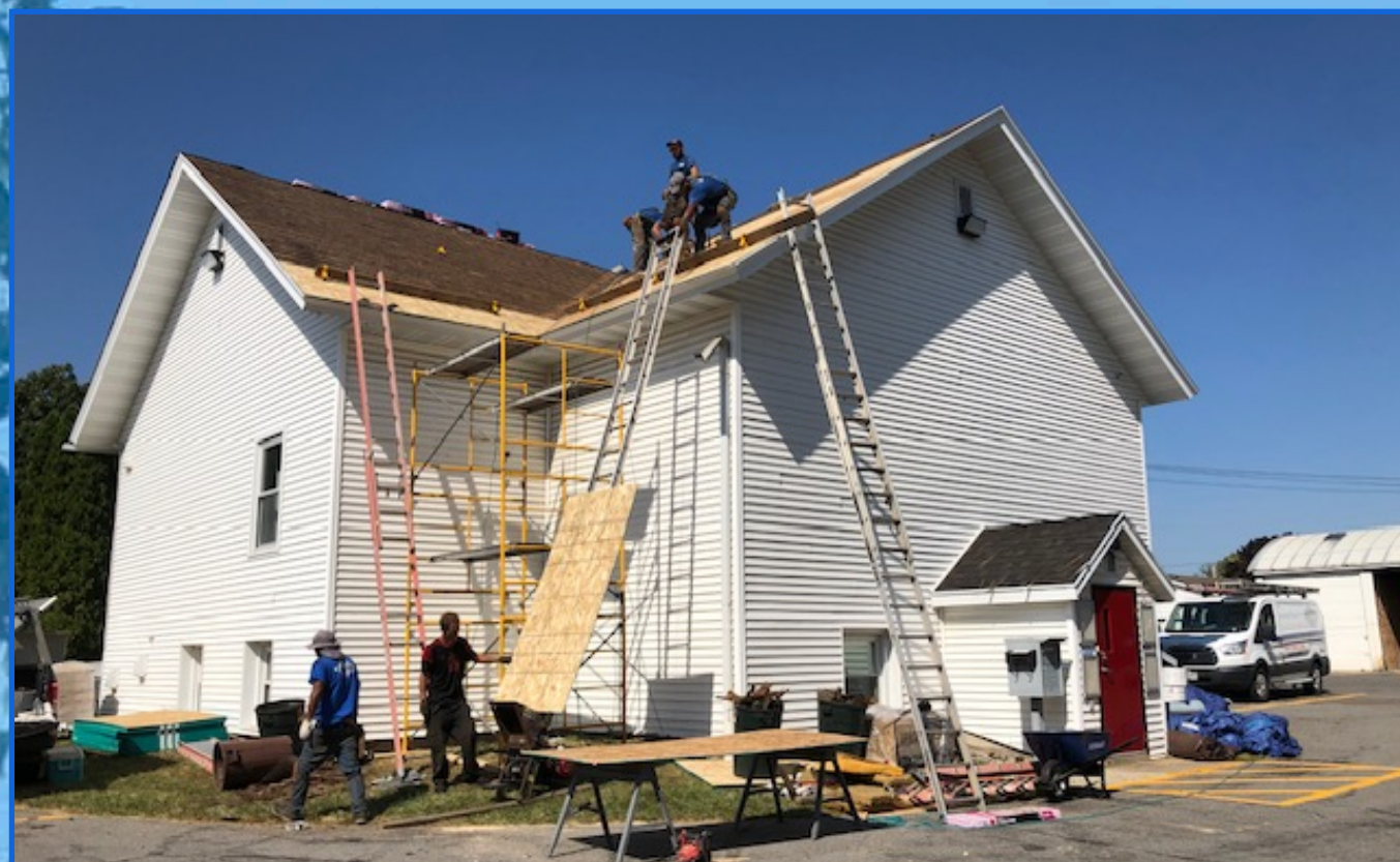
Roof replacement Sept. 2024
